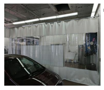
**Results:** Curtains are pulled out to seperate work areas. Chemicals and overspray are safely contained in the wash bay area.
